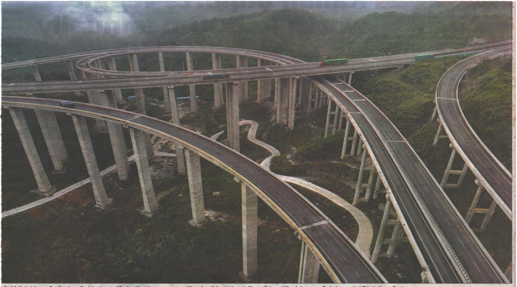
Aerial photo taken on Sunday shows the interchange of Baofu Expressway and Yongshun-Hepu Highway in Yunnan Tuli and Miao Autonomous Prefecture, central China's Hunan Province.
